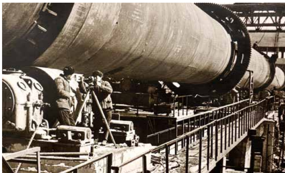
Sintering Furnace №8 Pavlodar Alumina Plant Aluminium of Kazakhstan JSC Pavlodar city
